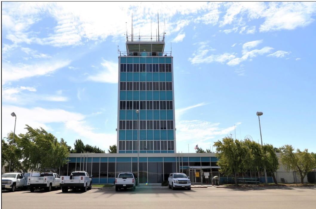
Photo 3: Northeast elevation, view southwest (9/11/23).
