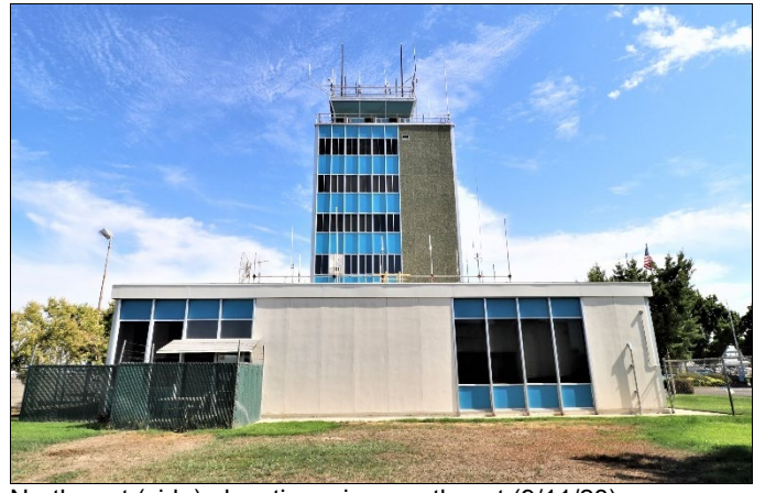
Northwest (side) elevation, view southeast (9/11/23).
