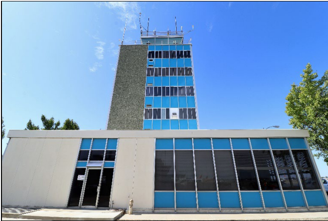
Southeast (side) elevation, view northwest (9/11/23).
