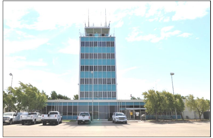
Northeast elevation, view southwest (9/11/23).
