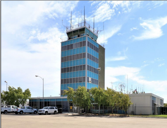
Northeast elevation, view south (9/11/23).
