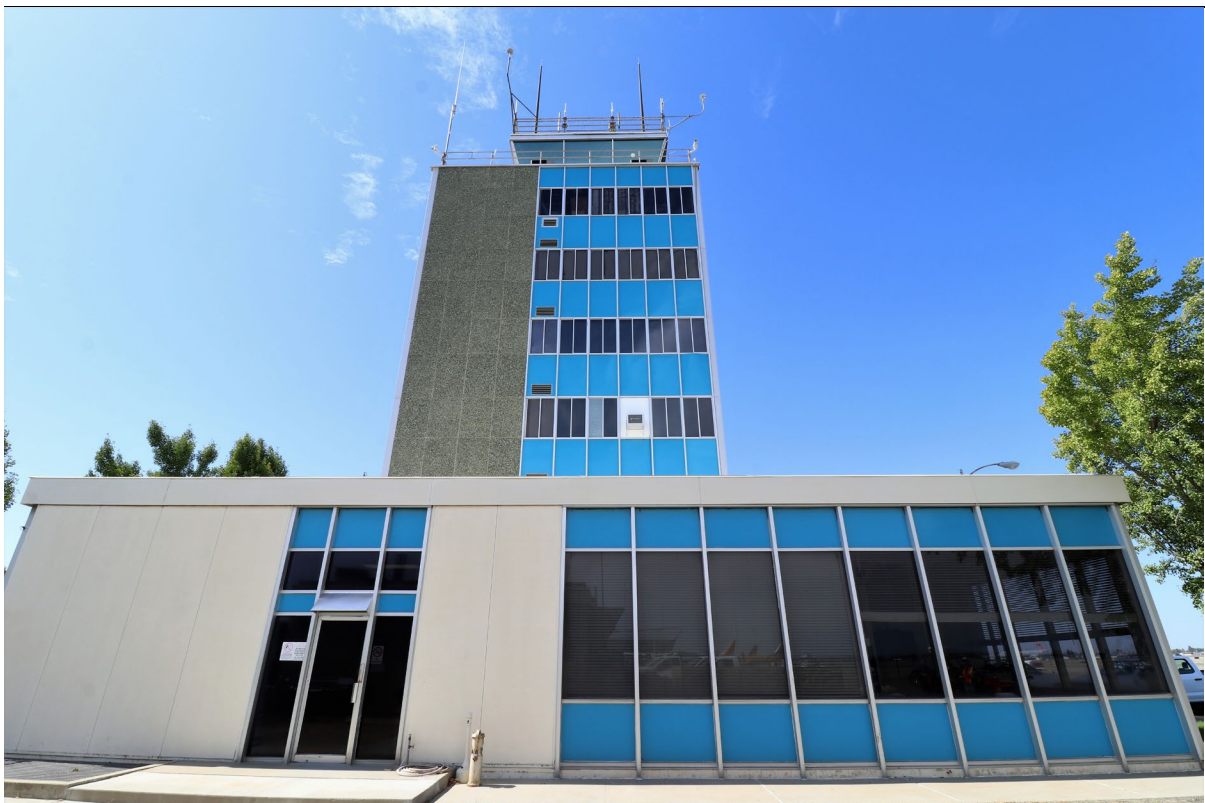
Photo 2: Southeast elevation, view northwest (9/11/23).
