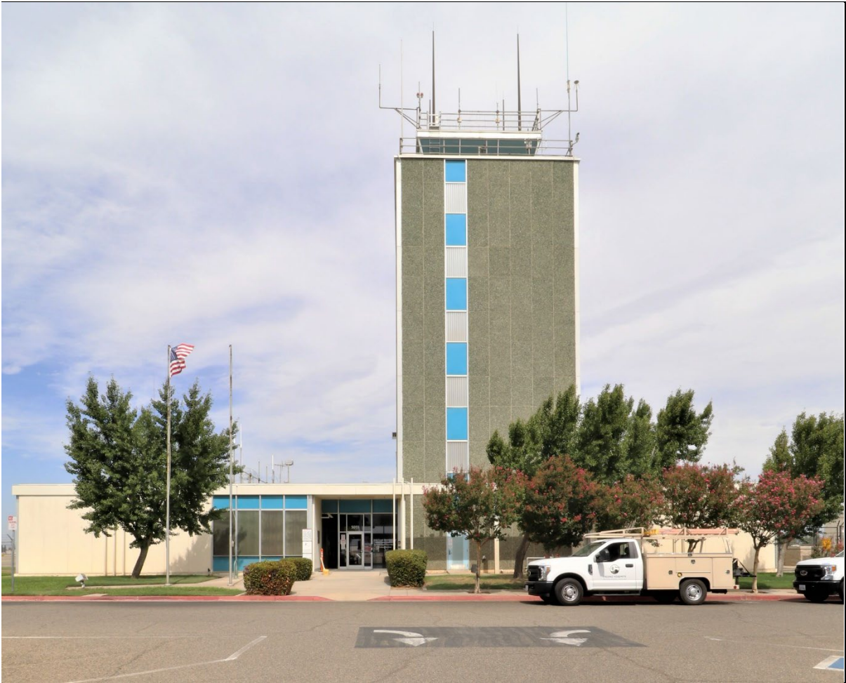
Photo 1: Southwest elevation, view northeast (9/11/23).
